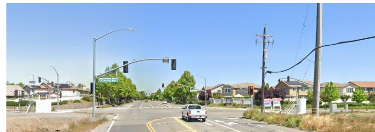
6. SR 113 at Parkway Blvd
