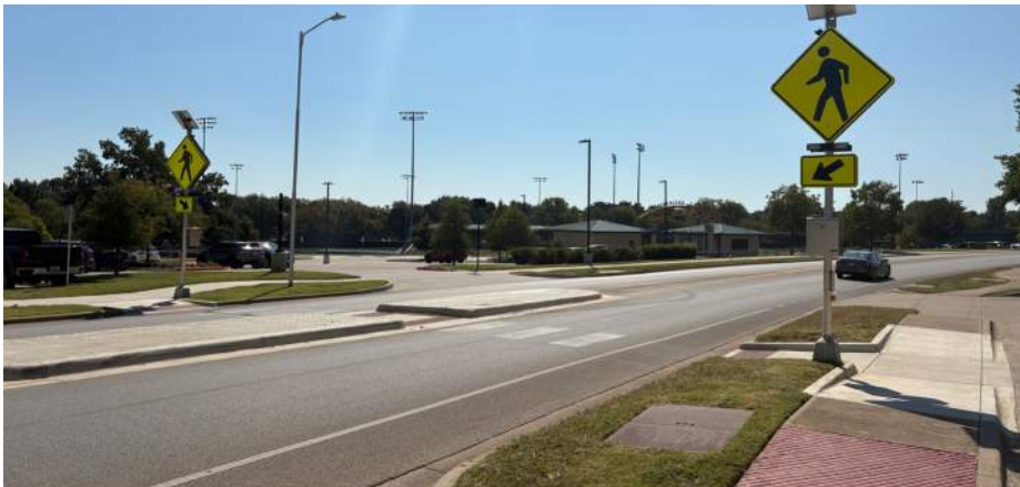
FIGURE 33: RECTANGULAR RAPID FLASHING BEACONS (RRFB)
