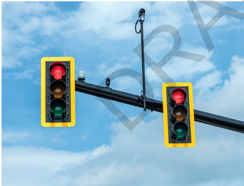
FIGURE 39. RETROREFLECTIVE BACKPLATES
