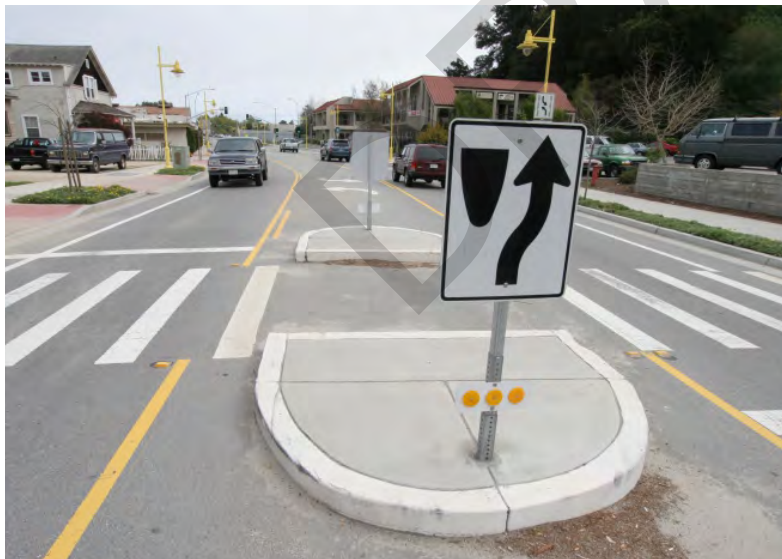
FIGURE 33. MEDIAN AND PEDESTRIAN REFUGE ISLAND
