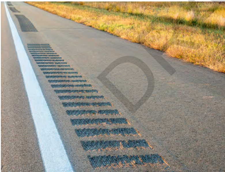
FIGURE 32. LONGITUDINAL RUMBLE STRIPS AND STRIPES ON TWO-LANE ROADS
