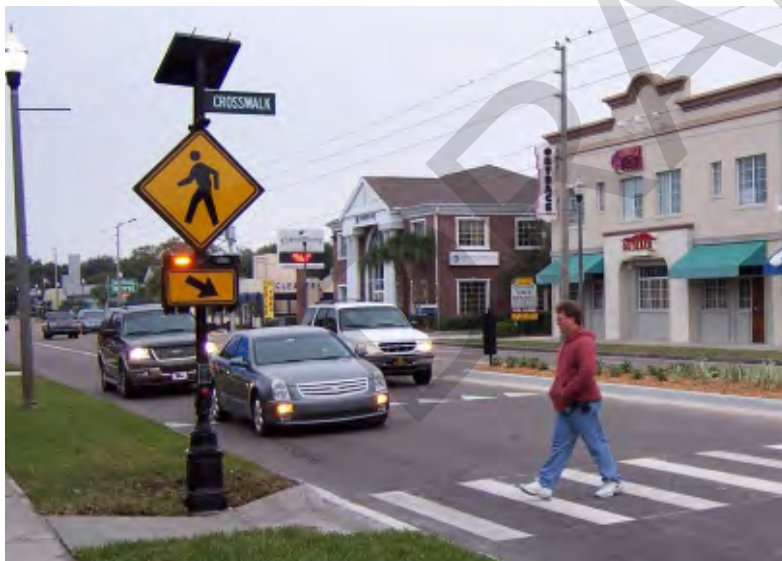
FIGURE 37. RECTANGULAR RAPID FLASHING BEACON
