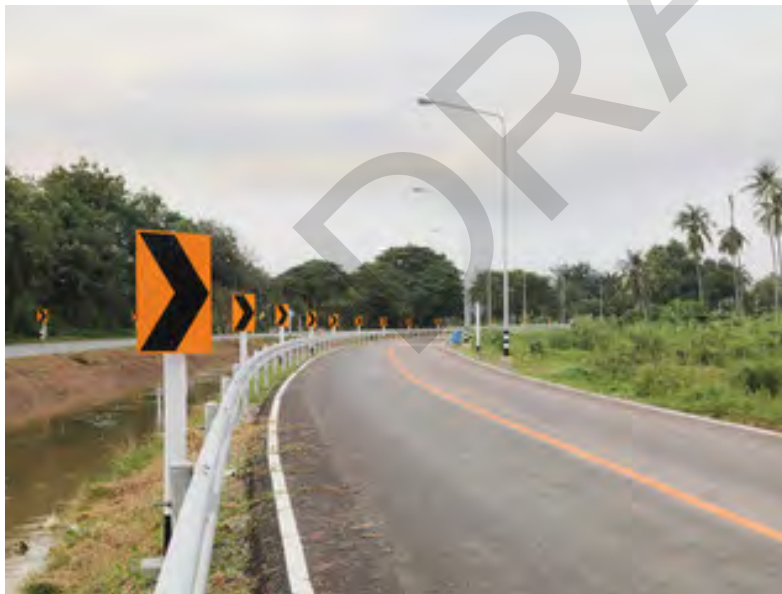
FIGURE 29. ENHANCED DELINEATION FOR HORIZONTAL CURVES
