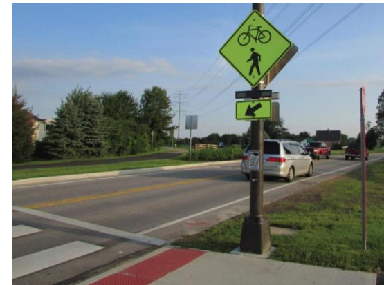
Rectangular Rapid Flashing Beacons
