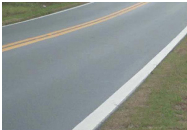
Figure 34. Wider Edge Lines
