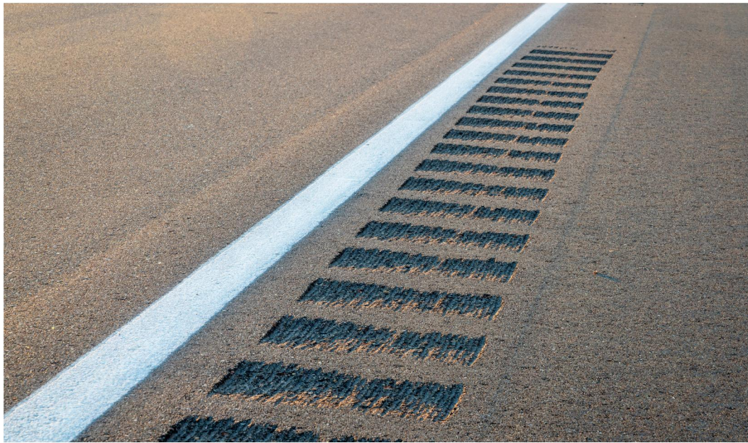
FIGURE 43. EXAMPLE OF LONGITUDINAL RUMBLE STRIP
