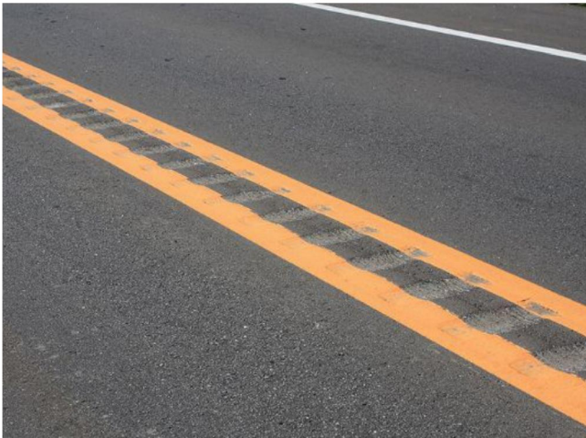
FIGURE 22. CENTERLINE RUMBLE STRIP
