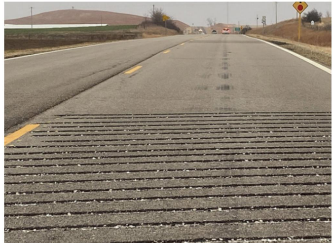
FIGURE 23. TRANSVERSE RUMBLE STRIP
