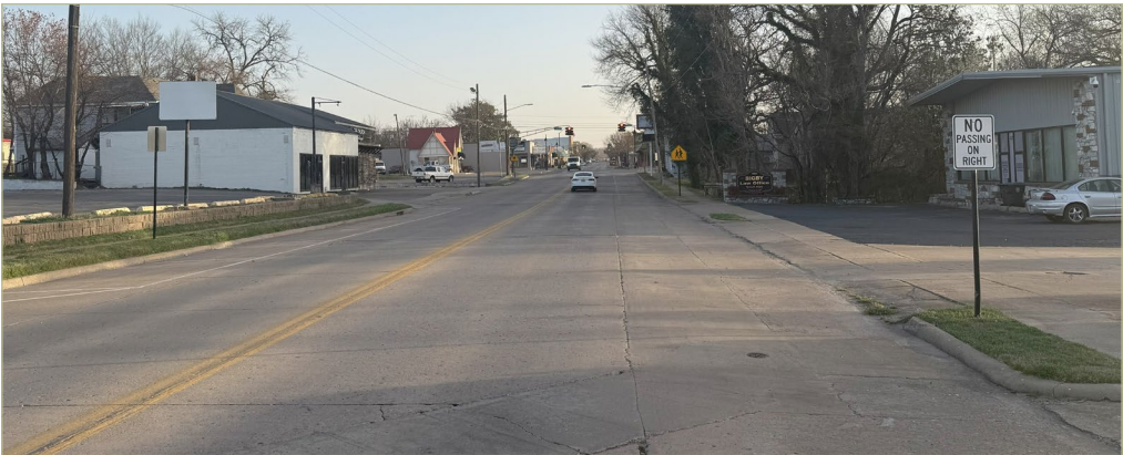
FIGURE 26. DRIVEWAY IN NEED OF CHANGE
