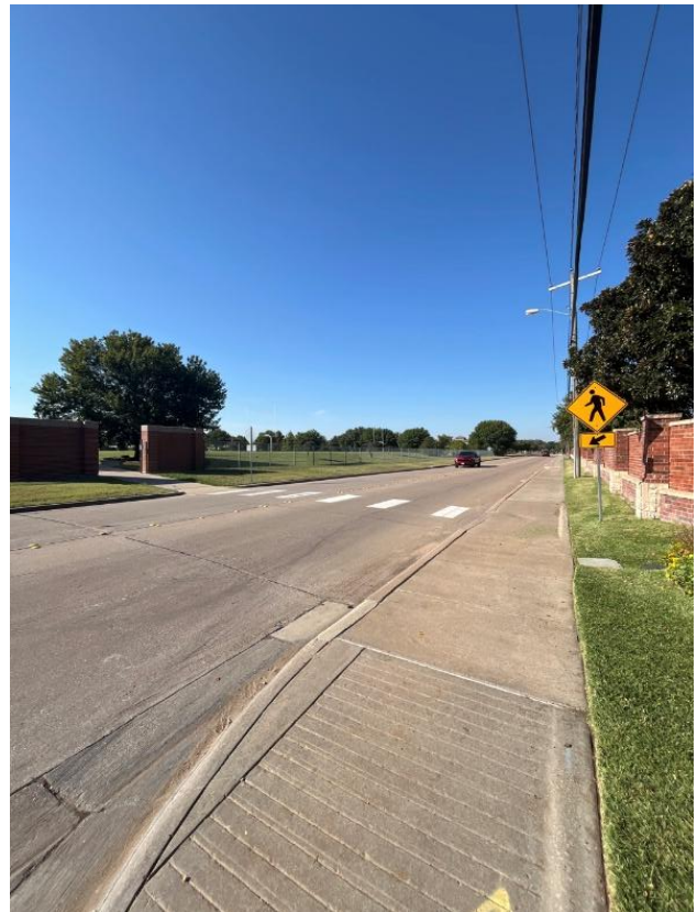
Figure 30. Upgrade to Rectangular Rapid Flashing Beacon
