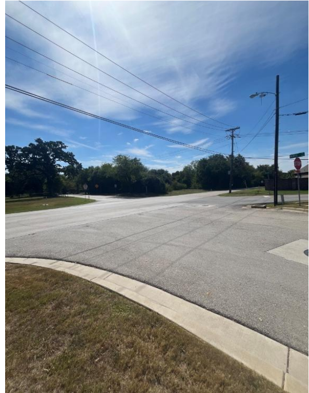
Figure 6. Full Signal Rebuild Needed, Upgrade Crosswalks, Directional Curb Ramps
