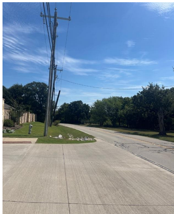
Figure 3. Sight Distance Issues Looking East
