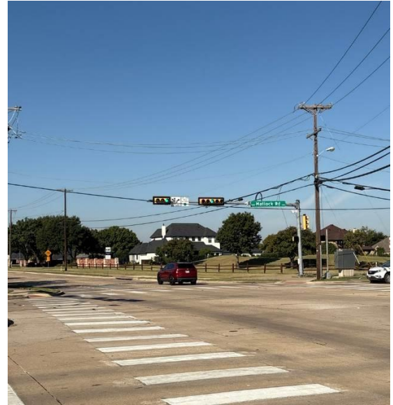
Figure 28. Flashing Yellow Arrow Needed
