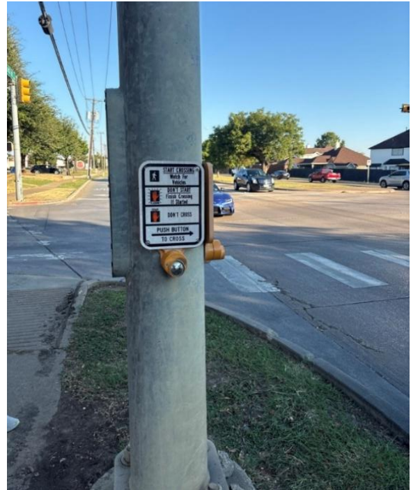
Figure 14. Update Needed to Pedestrian Push Buttons and Refreshing of Crosswalk
