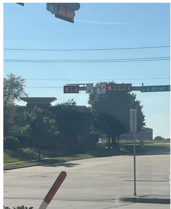
Figure 25. Upgrade Signage to Flashing Yellow Arrow
