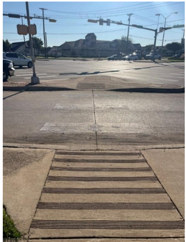
Figure 18. Detectable Surfacing Needed
