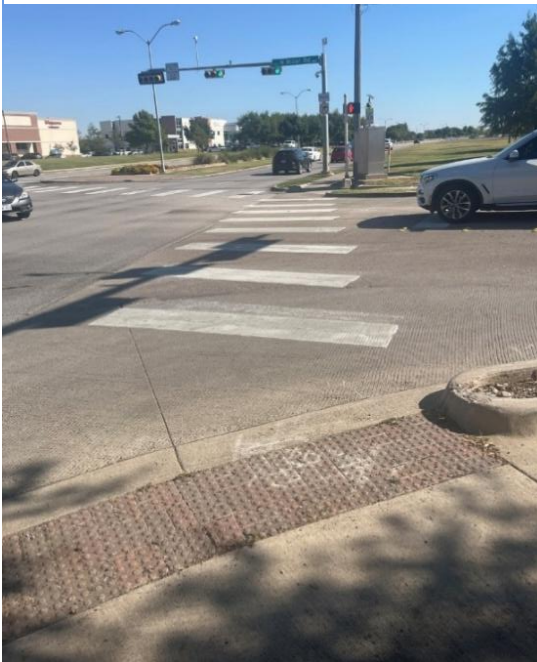
Figure 31. Upgrade to Directional Ramps
