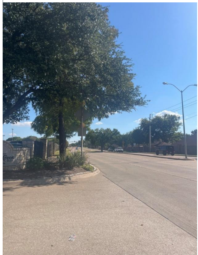
Figure 20. Recommended to Clear Trees to Improve Sight Distance
