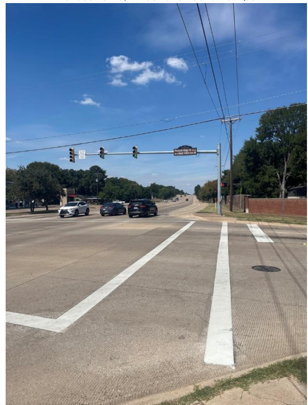
Figure 6. Full Signal Rebuild Needed, Upgrade Crosswalks, Directional Curb Ramps
