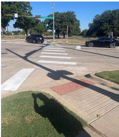
Figure 36. Upgrade Directional Ramps
