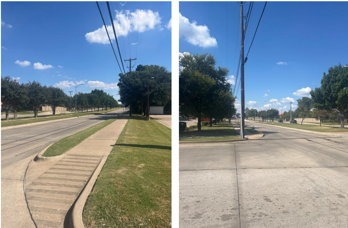
Figure 8. Poor Sight Distance Looking West – left; Looking East – right | Hooded Left Turn Recommended
