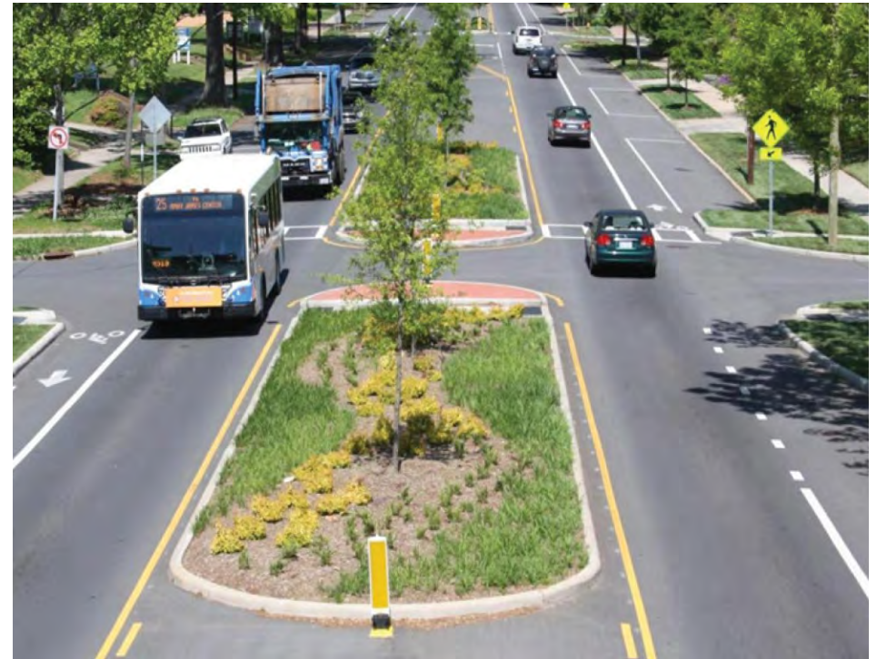
Figure 14. Raised Median Example
