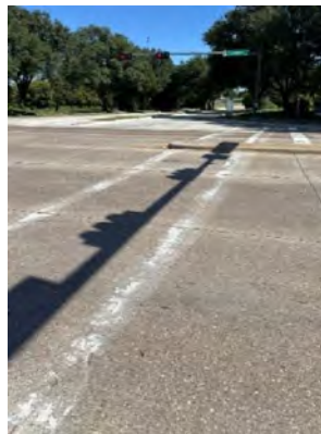
Figure 7. Median Nose Extends Past Existing Crosswalk
