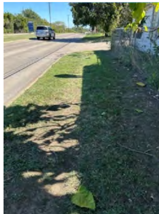
Figure 4. Example of Existing Worn Pedestrian Paths within the Parkway
