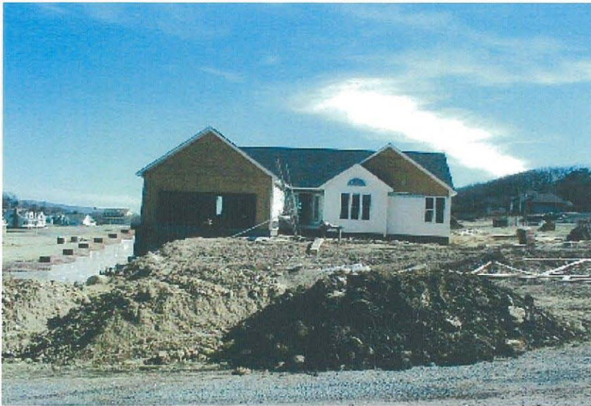
Photo 6.1 New Housing Construction
