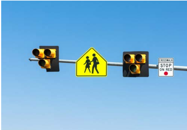
Figure 26. Pedestrian Hybrid Beacon
